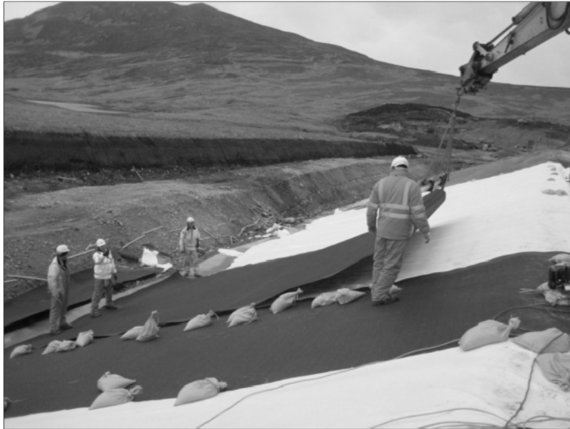
Figure 7. Photograph of Upstream Toe Plinth and Geomembrane
